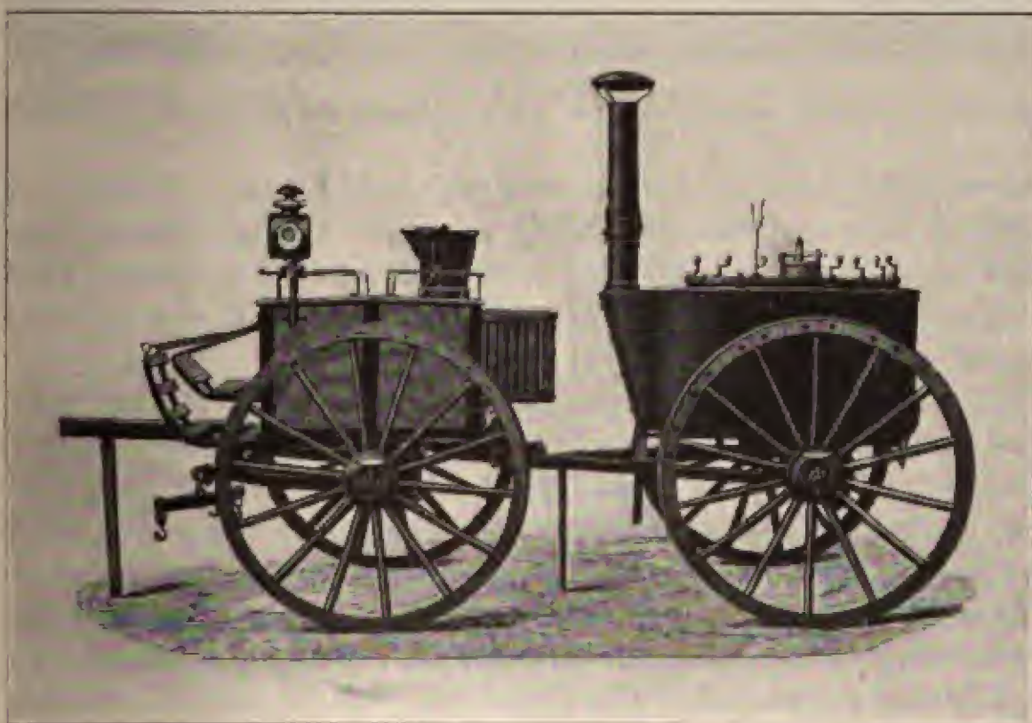
FIG. 81.— Russian wheeled kitchen for a company of infantry in the field.
